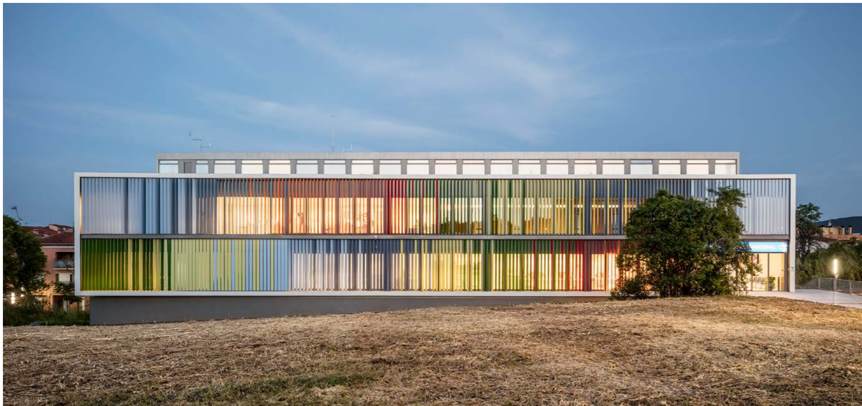
SOLAR PROTECTION LOUVRES
